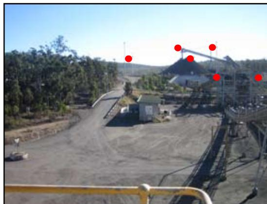
Actual wireless camera locations as shown by the red dots in this installation demonstrate the clear line of sight to the receivers where the picture was taken.
