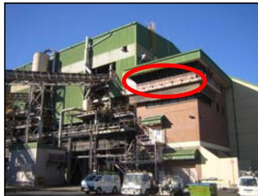
Receivers mounted at the control station are well above the ground plane to ensure there is no multipath interference.
